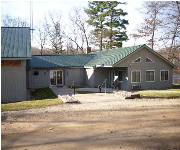
The new roof on the Clubhouse is now finished. It looks great and no more leaks.
